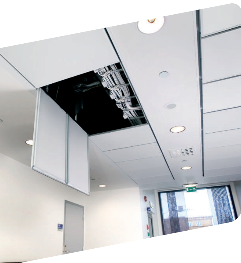
Fig. 1 - Installation of Hatch to Dry Wall
