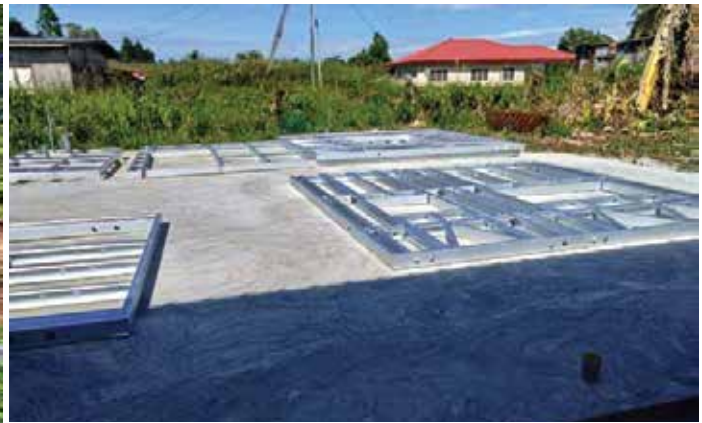
LGS frames at site ready to install
