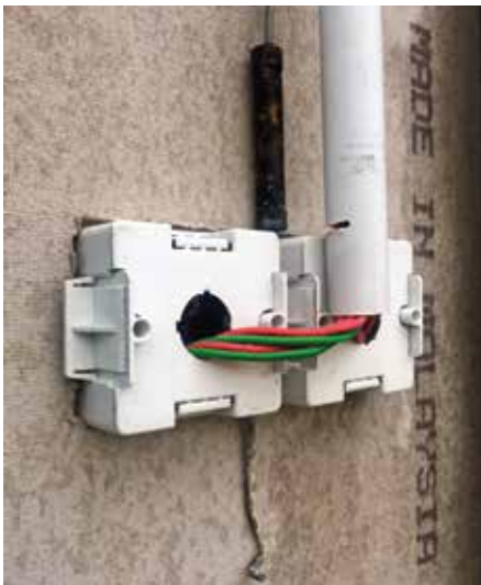
Use of specific 'clip-on' power socket (embedded type) for drywall (optional)
