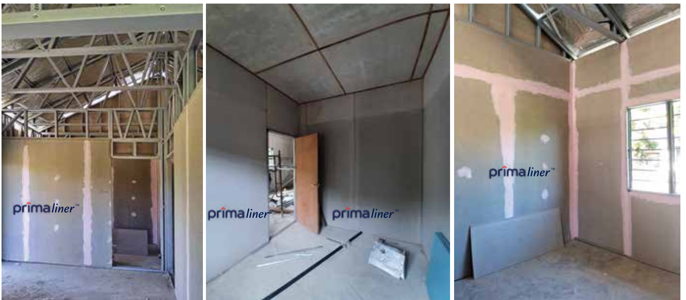
PRIMA Liner as interior walls
