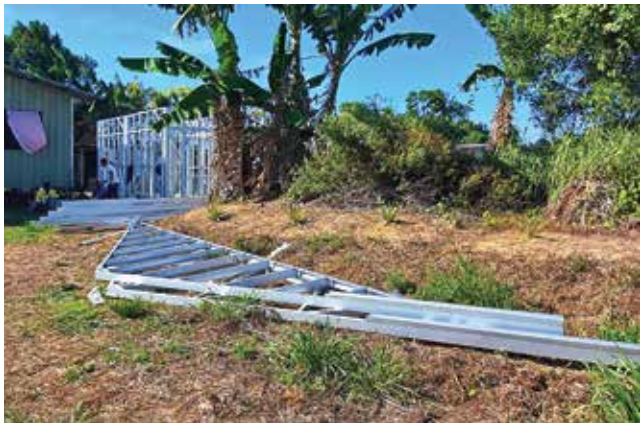
LGS frames at site
