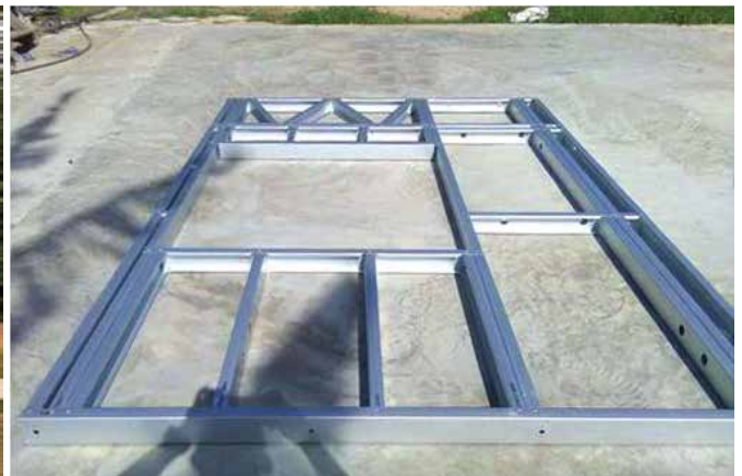
LGS Frame before installation
