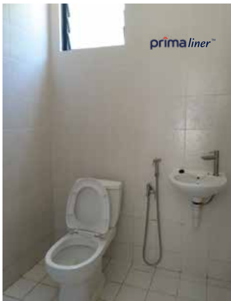
Tiles on PRIMA Liner wall
