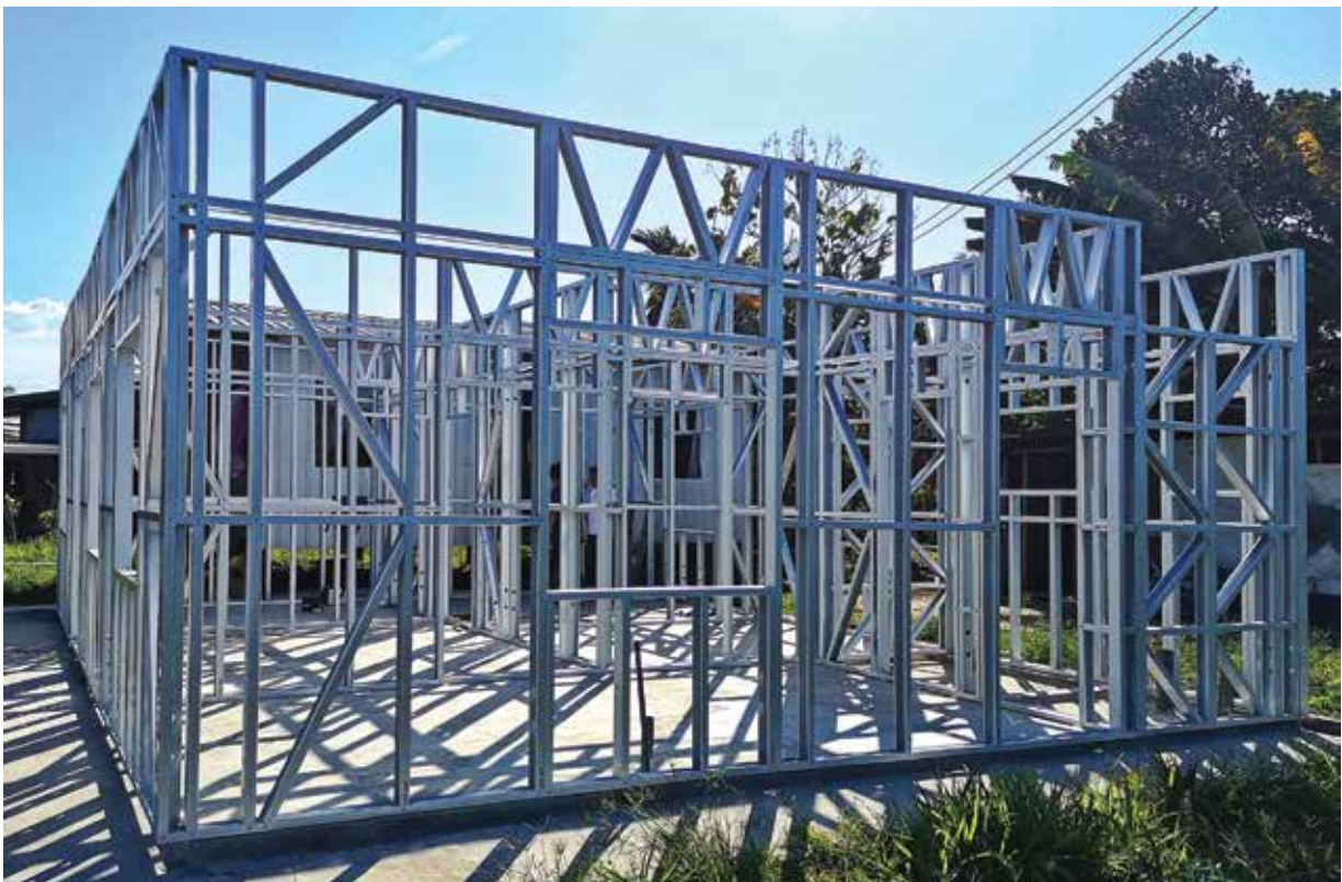
LGS Frames Structure
