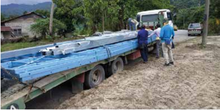
LGS frames deliver to site in bundle
