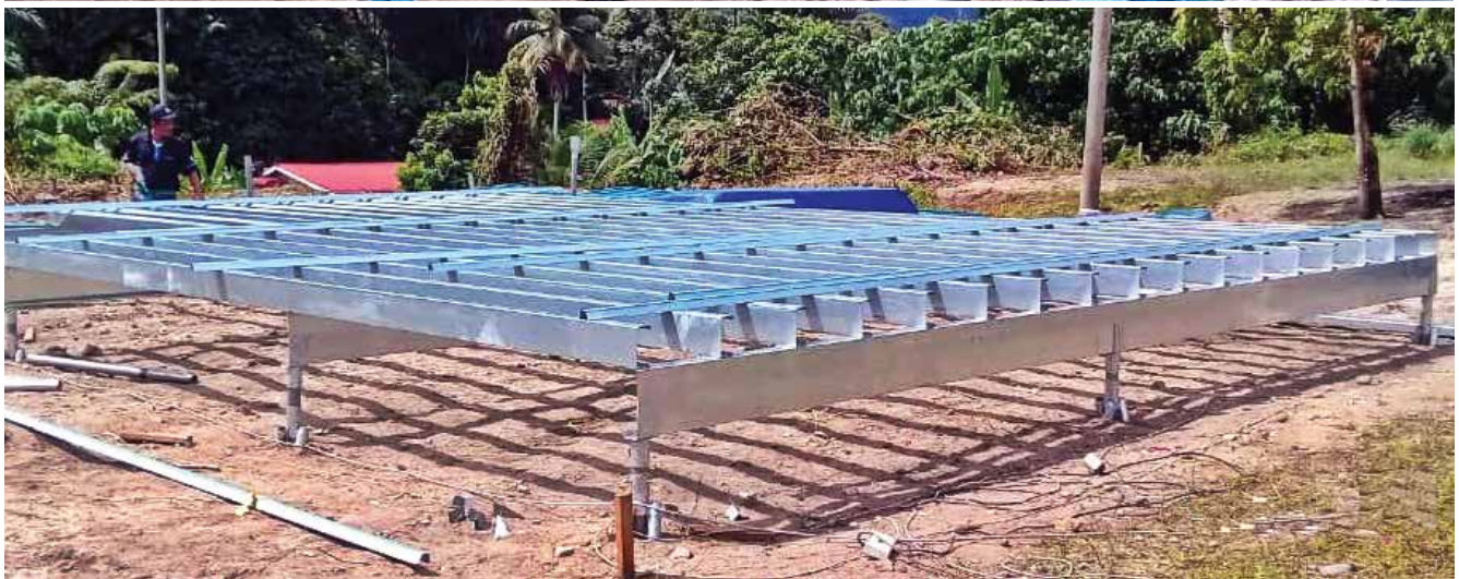
IBS Proprietary Anchorage System for elevated house
