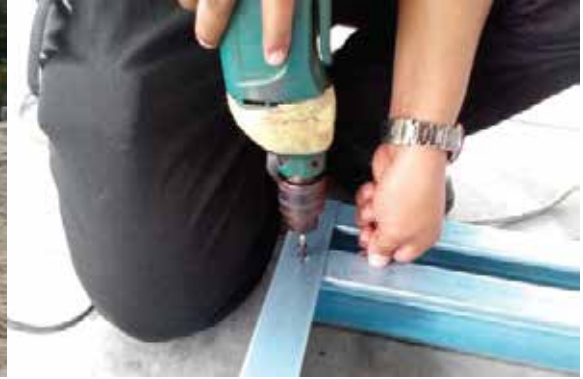
LGS frame installation using electric drill
