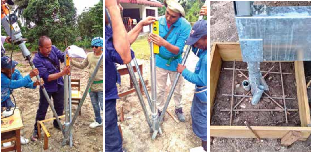
Tri-pod concept of soil anchoring
