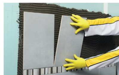
Tile onto Building Board
