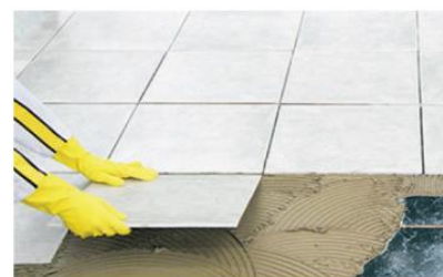
Tile onto Existing Tile
