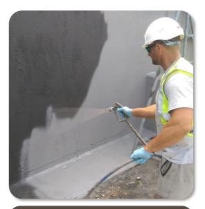
Liquid Applied Waterproofing Preformed / Sheet Waterproofing Membrane Integral Waterproofing
