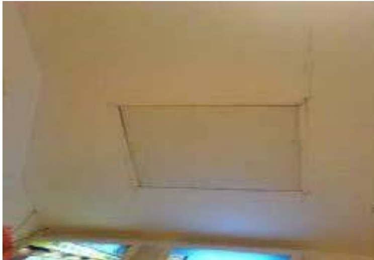
Poor Access Panel Detailing
