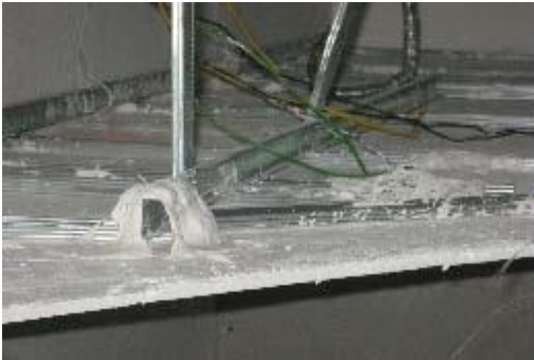
• Plaster Glass Material jointing with grouting (Mixture with fibre glass and gypsum)
