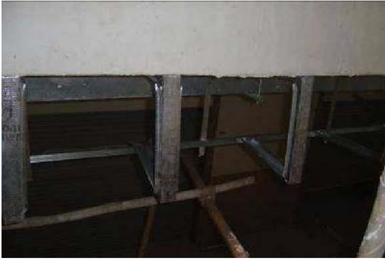
• Poor Bulkhead / L-Box Detailing
