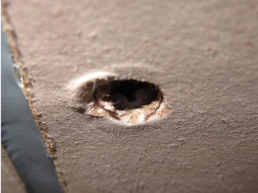
Deep Screw Fixing
