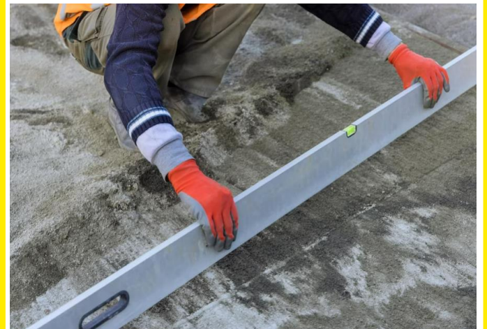
4 | Checking level of substrate surfaces
