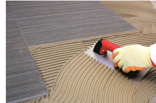
Improvisation of the Ceramic Tile installation method: Troweling System
