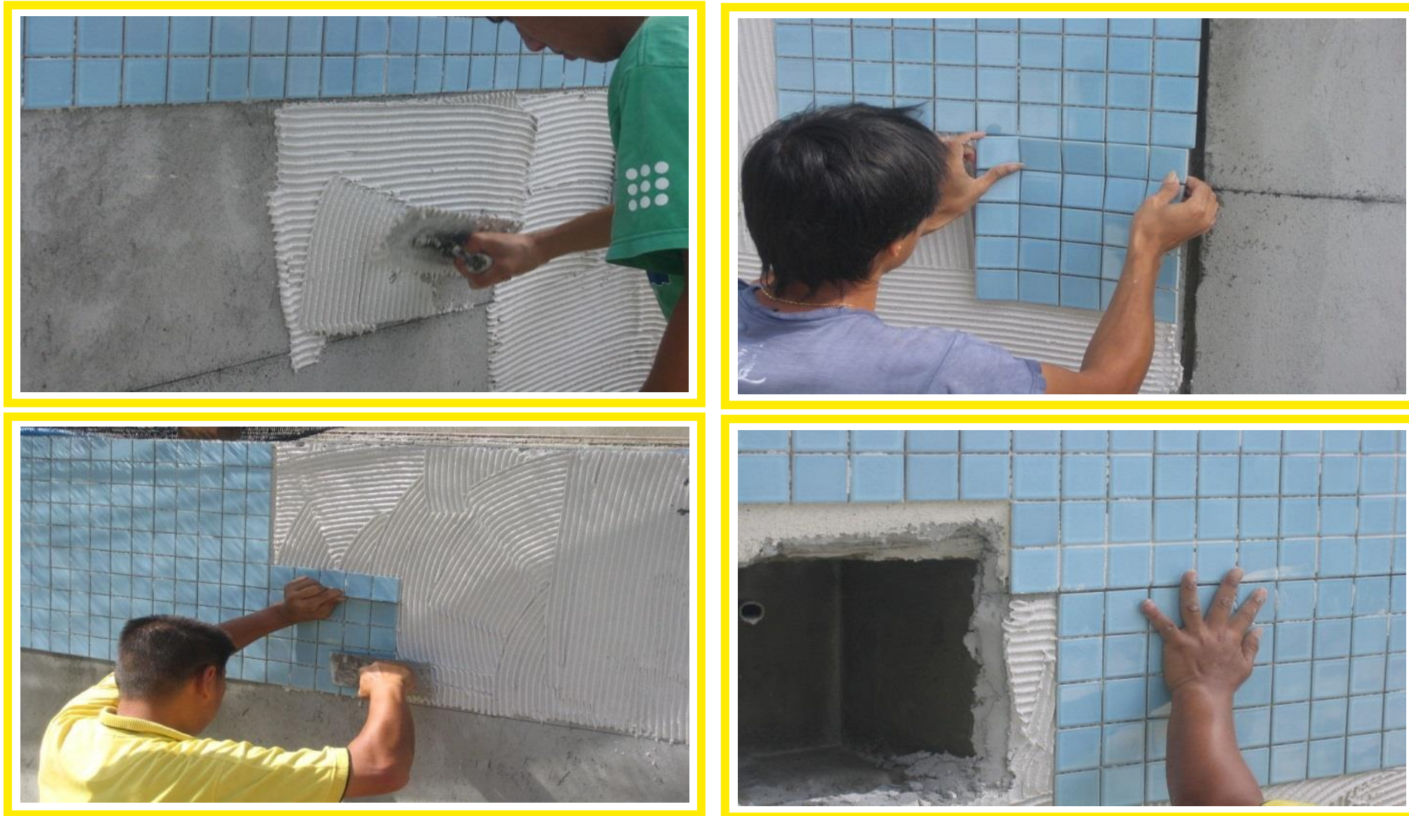
Fixing of Ceramic Mosaics To Swimming Pool
