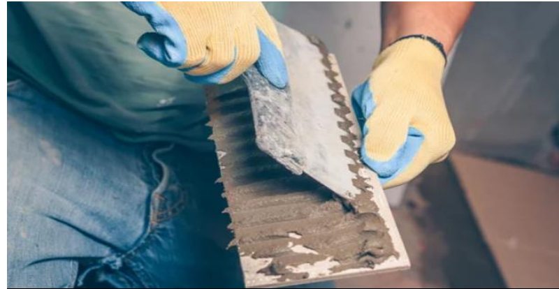
2 | Applying coat of mix on back surface of tile/ stone
