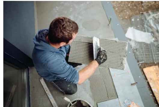
Tiles installed using Buttering system
