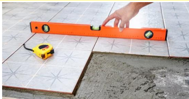
4 | Checking level of tile/ stone with spirit level
