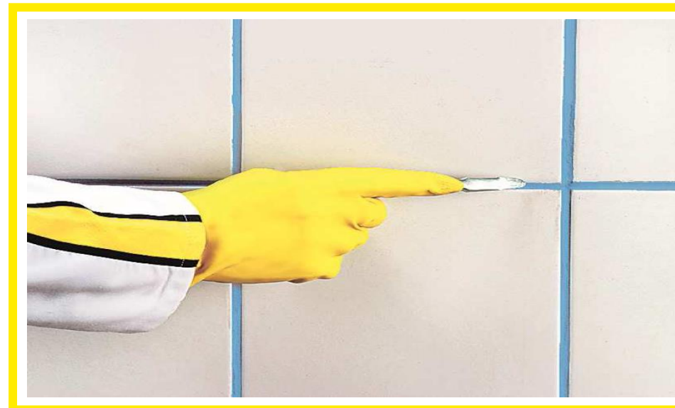
Cementitious Grouting of Ceramic Wall Tiles
