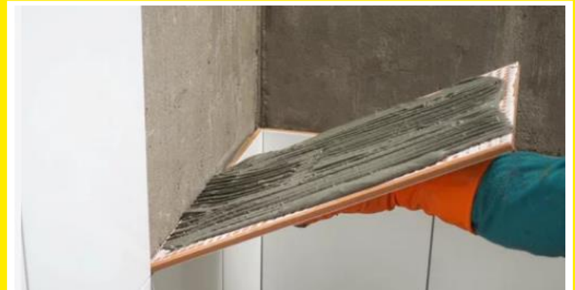
6 | Turn over tile/ stone to ensure satisfactory coverage of bedding
