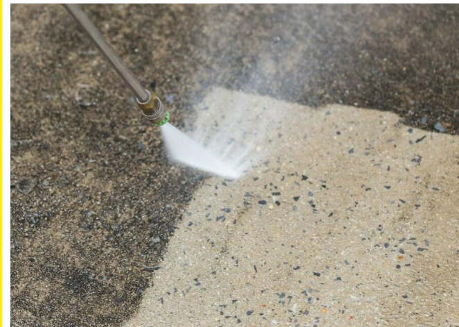
3 | Clean surface using water jet
