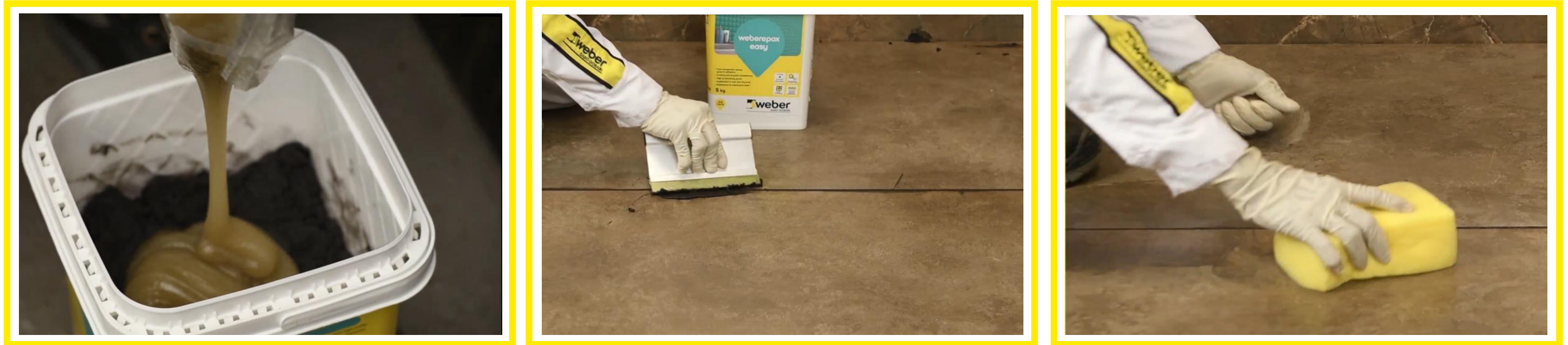
Epoxy Resin-Based Grouting System
