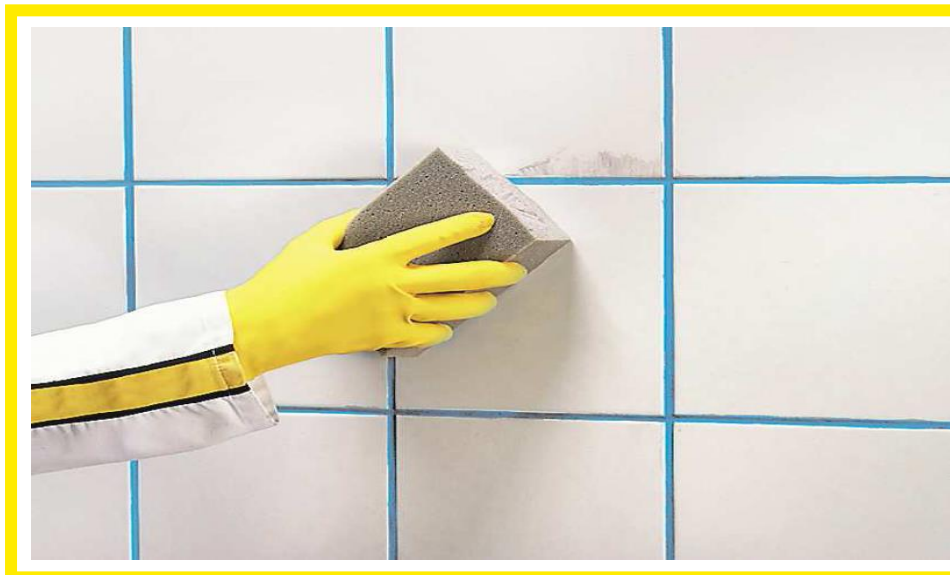
Cementitious Grouting of Ceramic Wall Tiles
