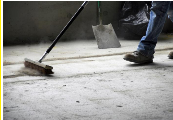
2 | Cleaning concrete surface with broom
