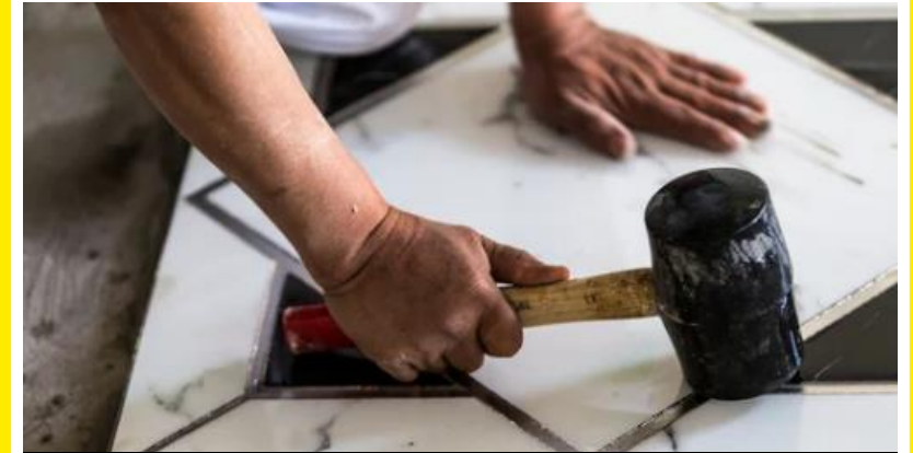
3 | Tapping tile/ stone onto uniform position
