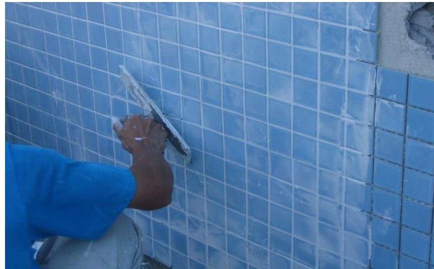
Latex Modified Grouting System To Swimming Pool
