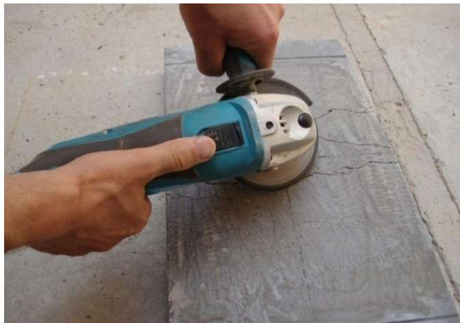
1 | Removing concrete protrusion
